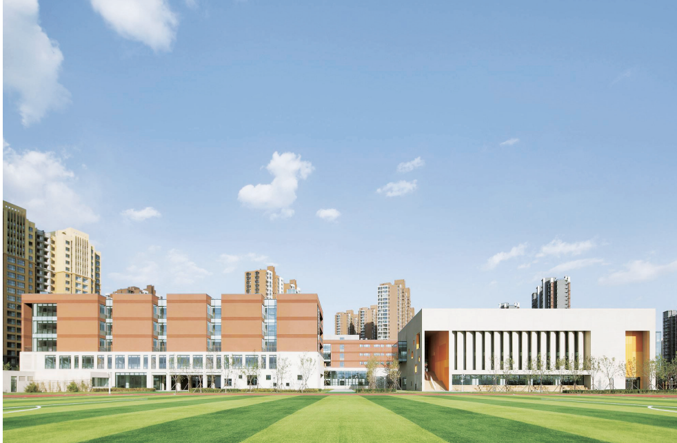
Beijing HuiLongGuan Middle School - 1 set of Medium Modular Data Center
