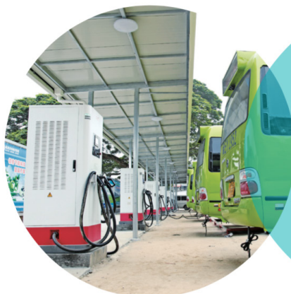
Zhangzhou Bus Station
