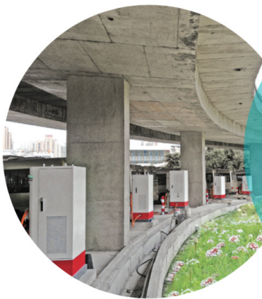
Ningde Bus Station
